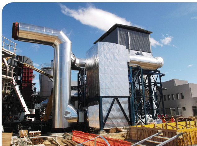
A Redecam DeNOx SCR system, able to achieve up to 95% \text{NO}_x reduction, with a bypass.
