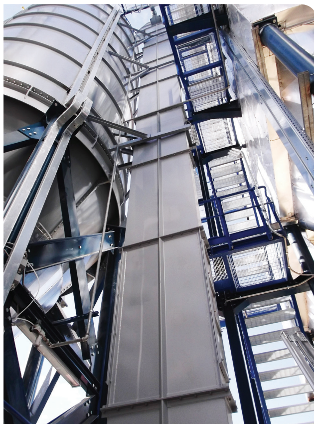
DID with in-duct lances is an ideal \text{SO}_x removal solution for retrofits, as it allows plants to keep existing air filtration and ancillary equipment.
